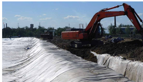
Anchorage of Mirafi® geotextile panel around periphery of sludge pond
