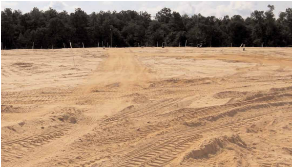
Completion of fill closure
