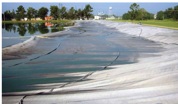
Pulling Mirafi® geotextile reinforcement panel across surface of sludge pond
