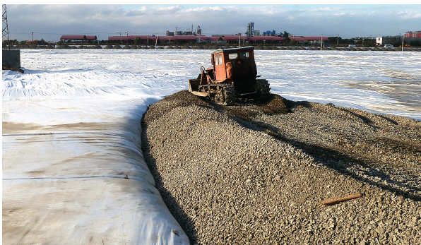
Constructing parallel fill fingers to stress Mirafi® geotextile reinforcement panel
