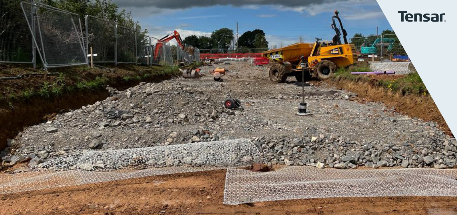
Single MSL (mechanically stabilised layer) delivering a bespoke solution and significant savings
