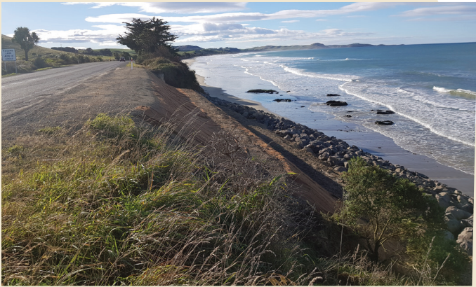
Road view after project completion
