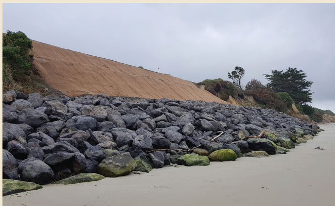
Beach view after project completion
