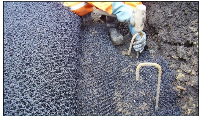
Fixing MacMat in trench
