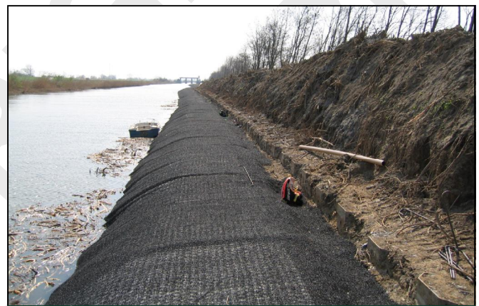
MacMat® R erosion protection on river bank
