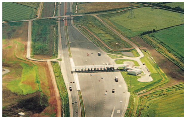
Second Severn Crossing Bridge Toll Plaza supported on Tensar geogrid LTP (UK).
