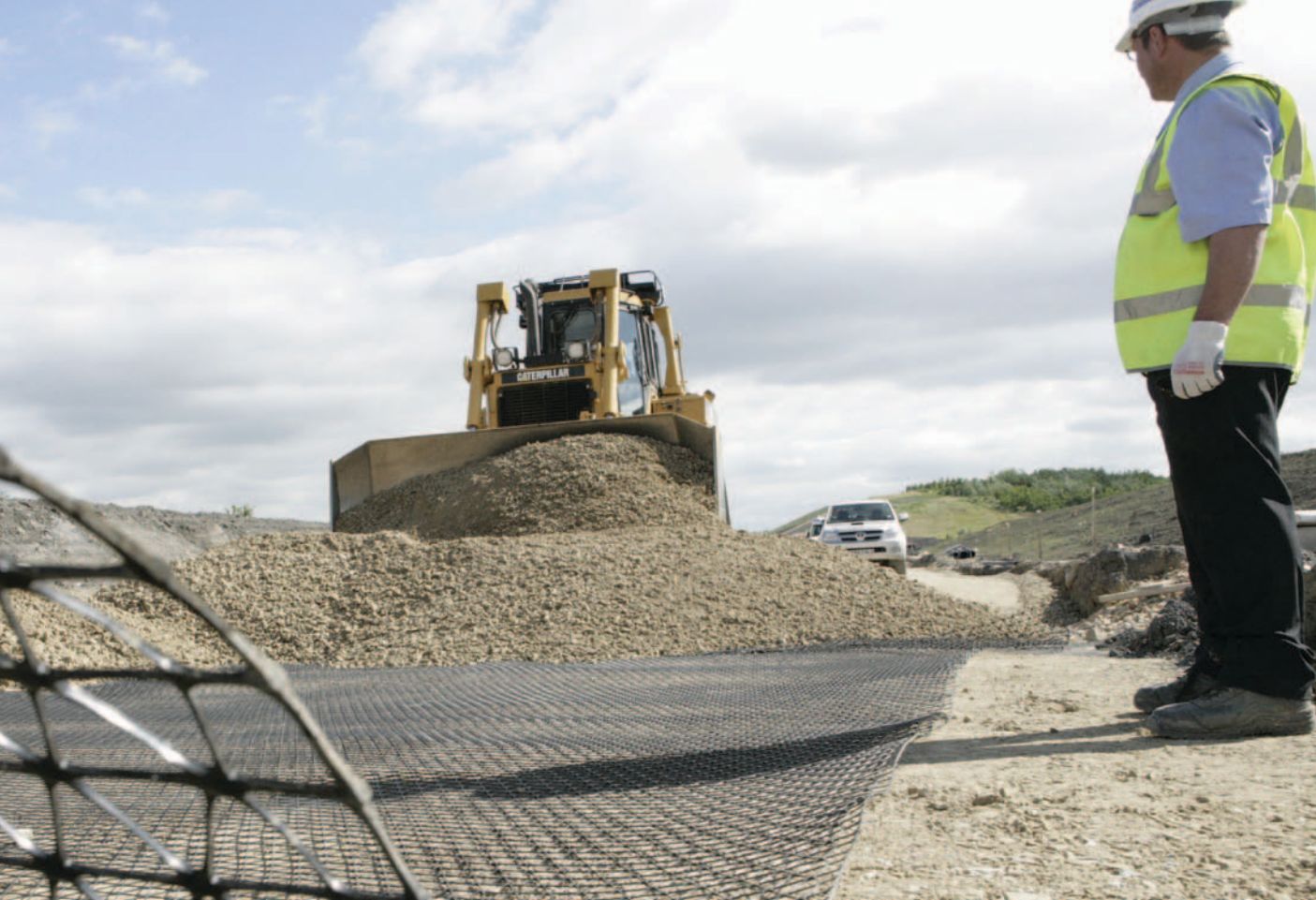
TriAx® gives improved aggregate confinement and interaction, leading to improved structural performance of the mechanically stabilised layer.
