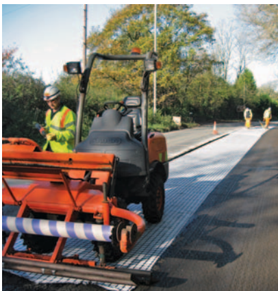
AR-GN bonds well into the underlying surface.
