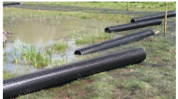
TriAx® gives improved aggregate confinement and interaction, leading to improved structural performance of the mechanically stabilised layer.
