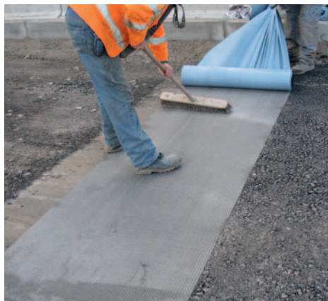
Glasstex®Patch™ 880 can be applied to most sound substrates utilising the adhesive coating.
