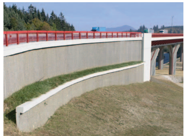
A variety of panels and finishes can be applied with either pre-cast or cast on-site panels.
