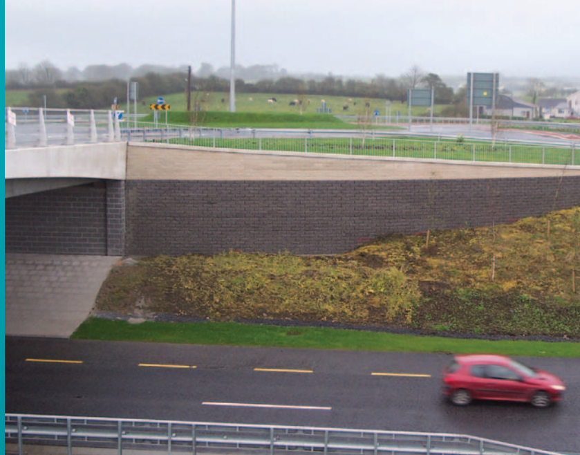
TensarTech Wall System – a combination of coloured facing blocks is used for dramatic effect on this bridge wingwall.
