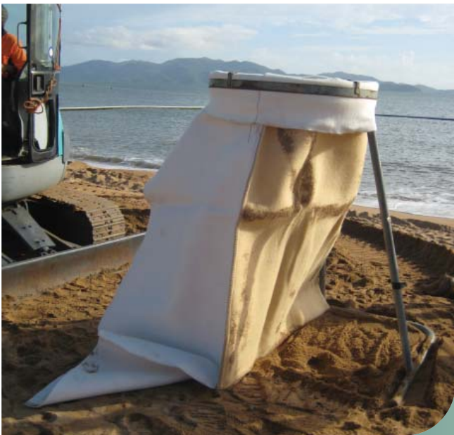
Figure 2. Securing sand container
