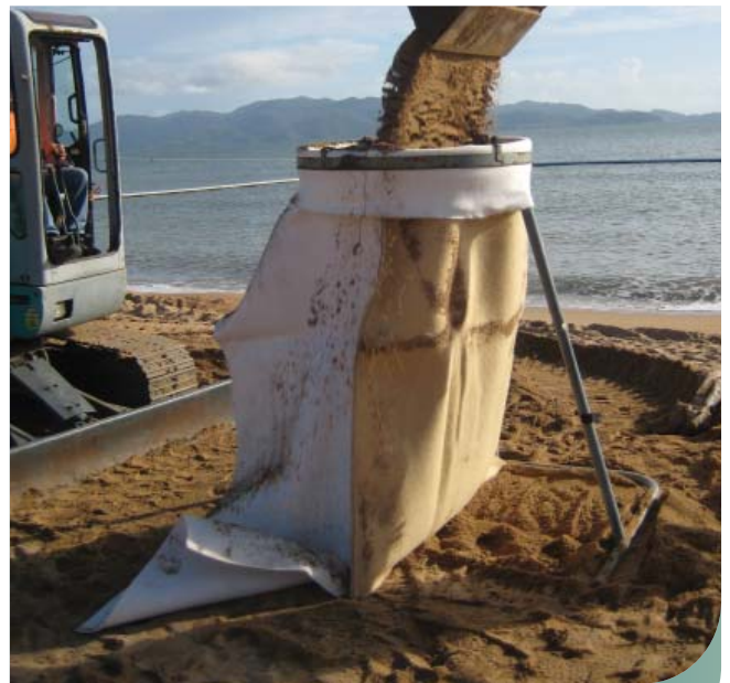
Figure 3. Filling sand container
