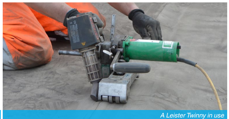
CC Hydro™ double/triple-track weld
