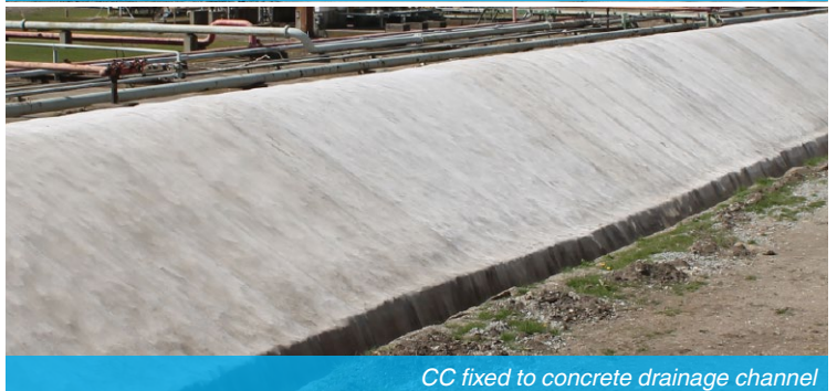
CC captured within a poured curb
