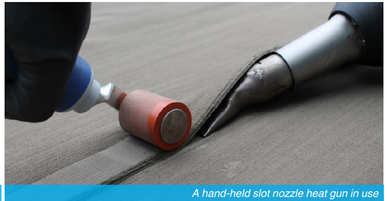
Thermally Bonded Overlap Joint
