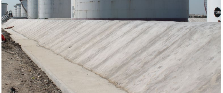
CC captured within a poured curb
