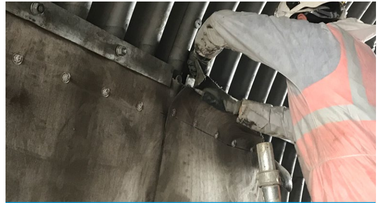
CC perimeter edge secured with clamping bar
