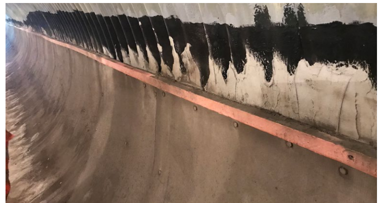
Timber secured to provide a cutting edge guide for a neat finish
