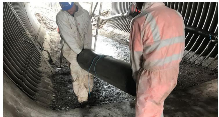
Bespoke batched CC transported into culvert
