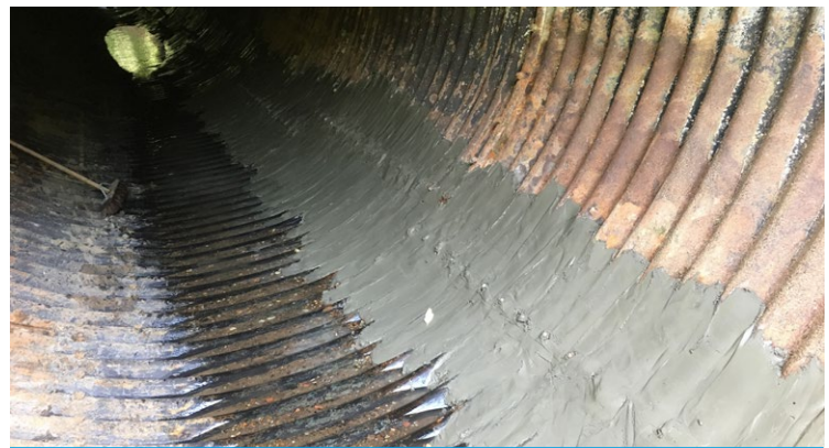
Smoothing over protrusions using grout
