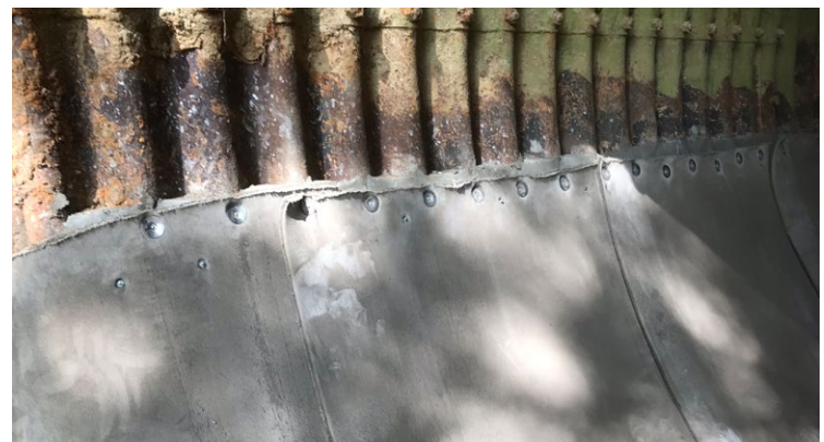
Perimeter edge secured with anchor fixings and washers
