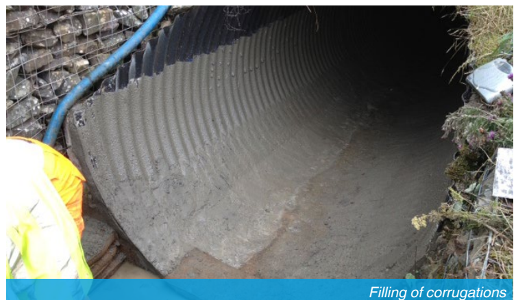
Smoothing over protrusions using grout
