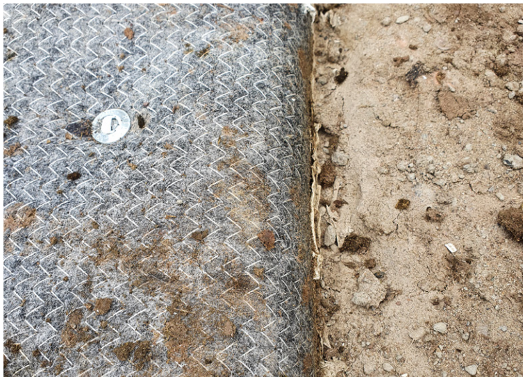
No evidence of scuffing, puncture or damage after 100 passes
