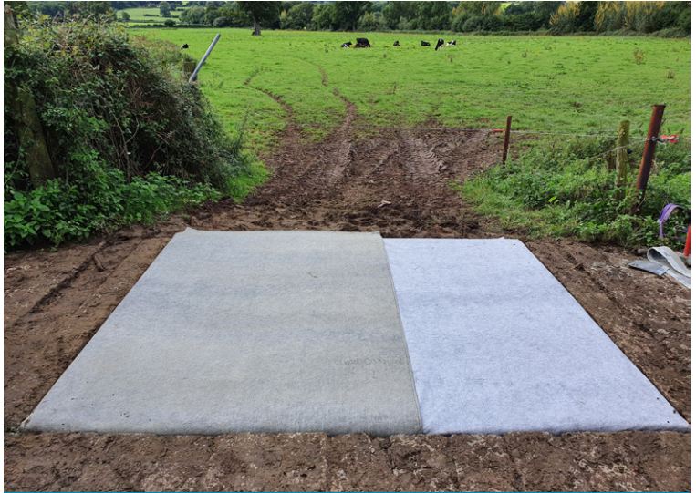
Installation of CCX-M™
