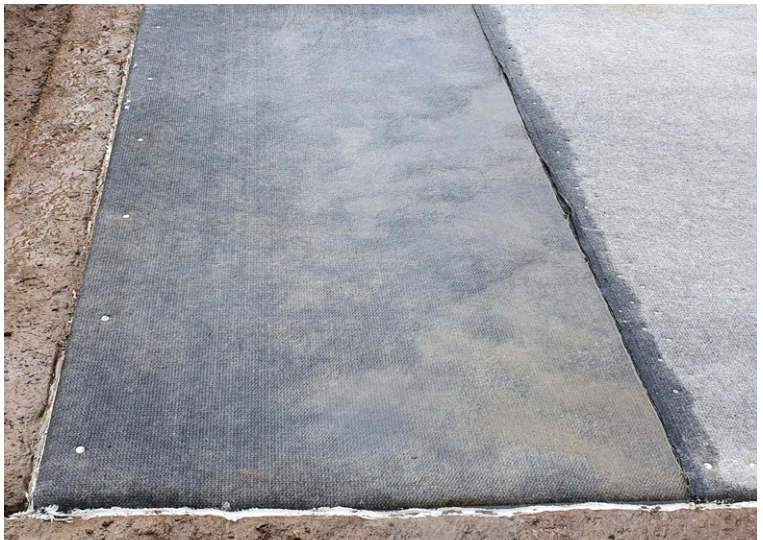
Overlap jointed and edges fixed to concrete sleepers below
