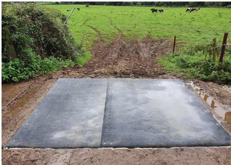
Installation completed and hydrated
