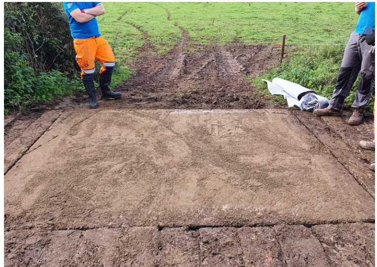
Sand screed layer
