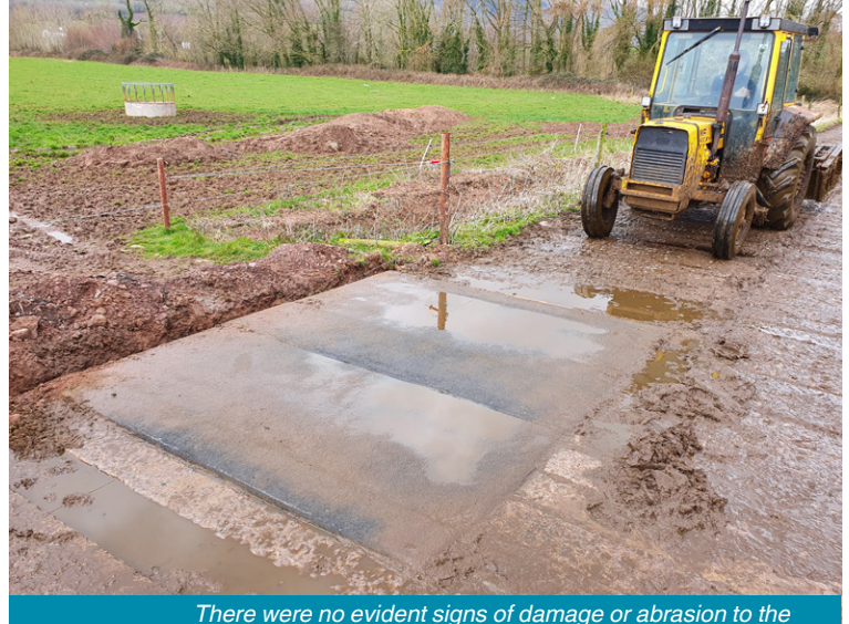
There were no evident signs of damage or abrasion to the
