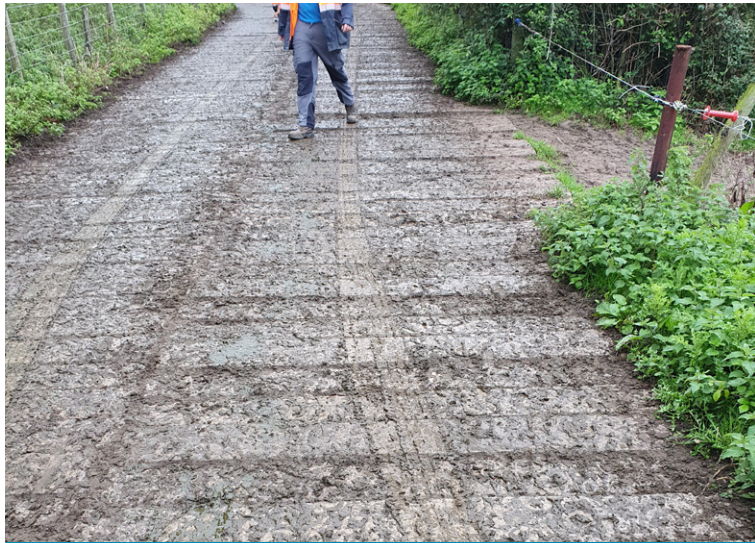
Site prior to installation
