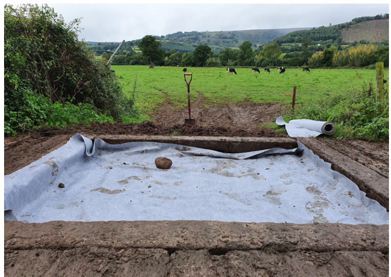
Installation of geotextile separation layer
