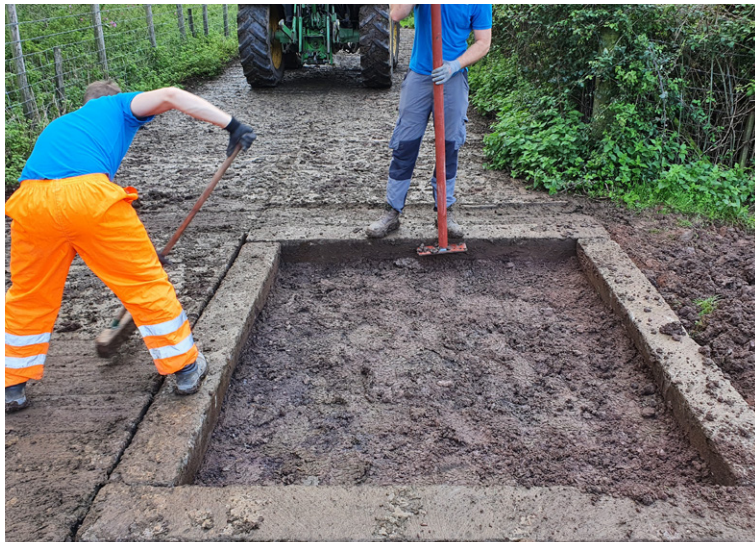
Realignment of outer sleepers and compacting substrate
