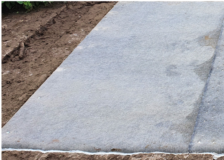
Edges sealed and underlap hydrated prior to jointing
