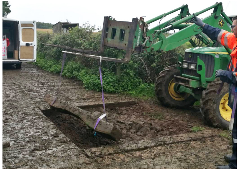
Removal of sleepers
