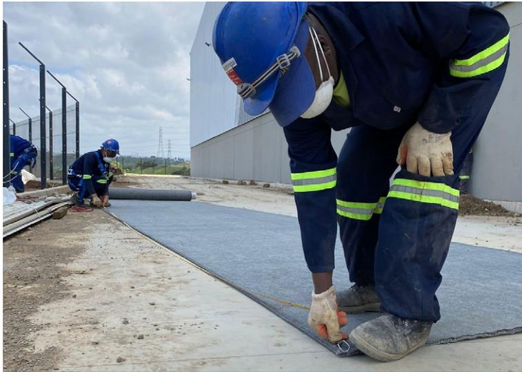
CCX-U™ measured before cutting and installing
