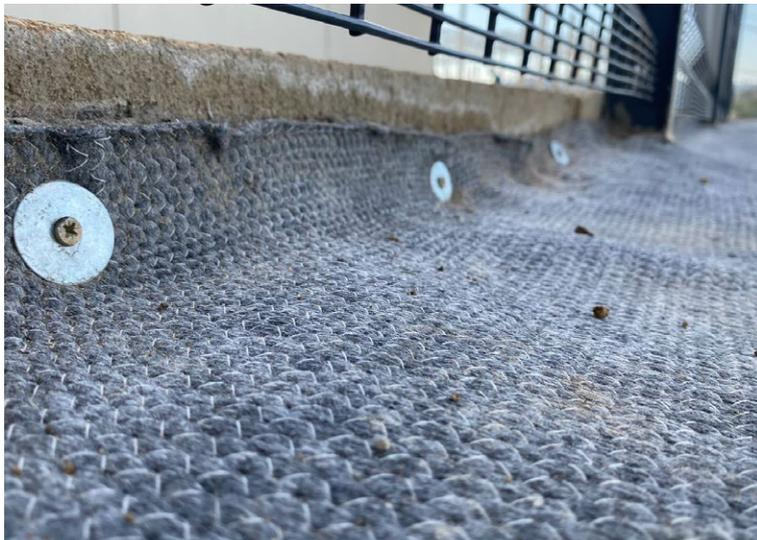
CCX-U™ fixed with 6x50mm masonry anchors
