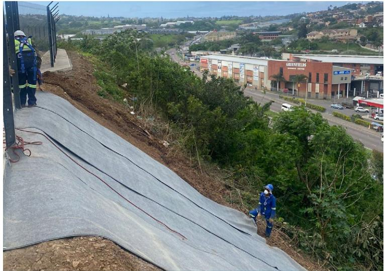
CCX-U™ Installed transversely down the slope
