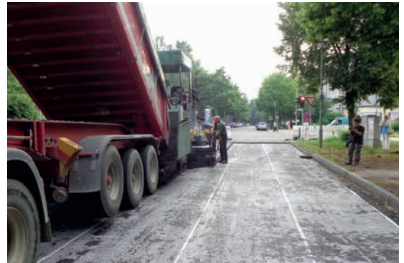
Pic. 9: Pave Overlay
