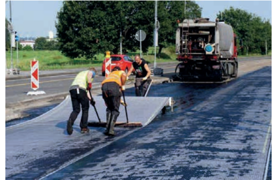
Pic. 5: Manual Installation of ADFORS GlasGrid
