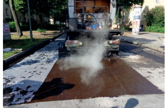
Pic. 3: Tack coat application before GlasGrid® CGL installation
