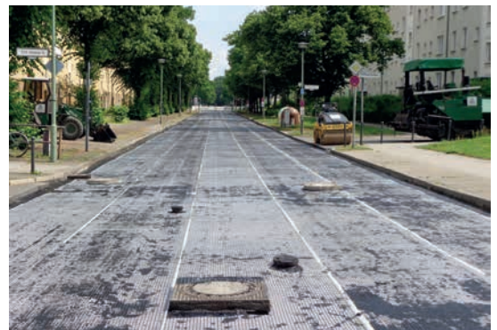
Pic. 2: Typical ADFORS GlasGrid CGL/ CG application on milled surface
