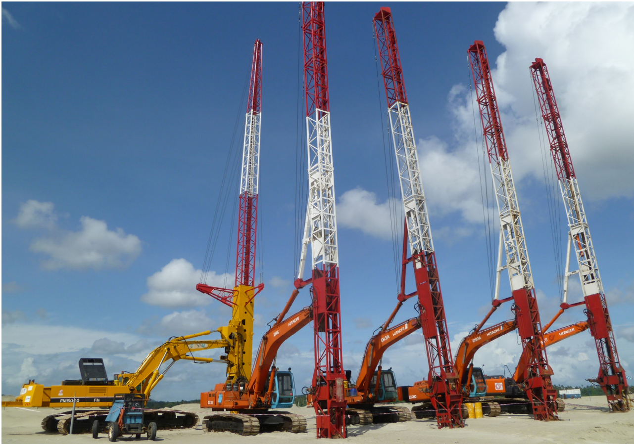
Prefabricated vertical drain installation rigs
