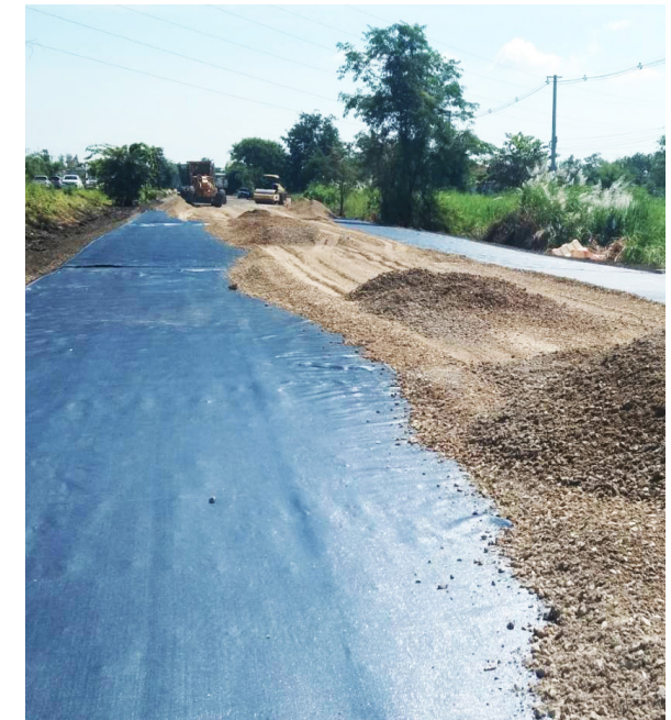
Pavement rehabilitation over expansive clay subgrade
