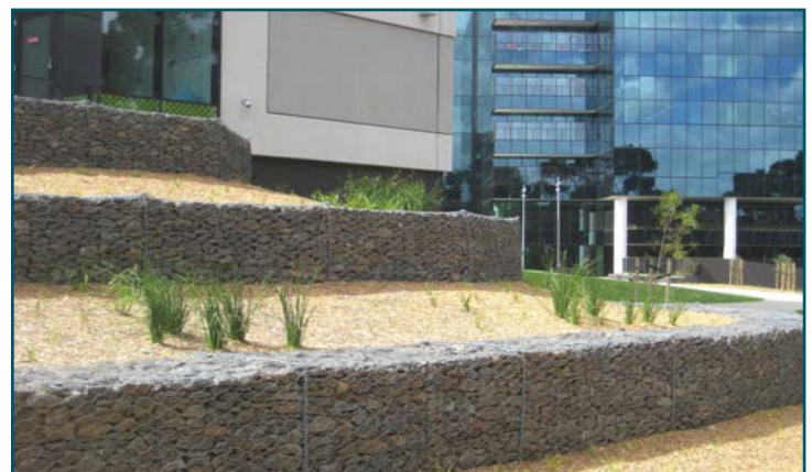
Typical Gabion Application
