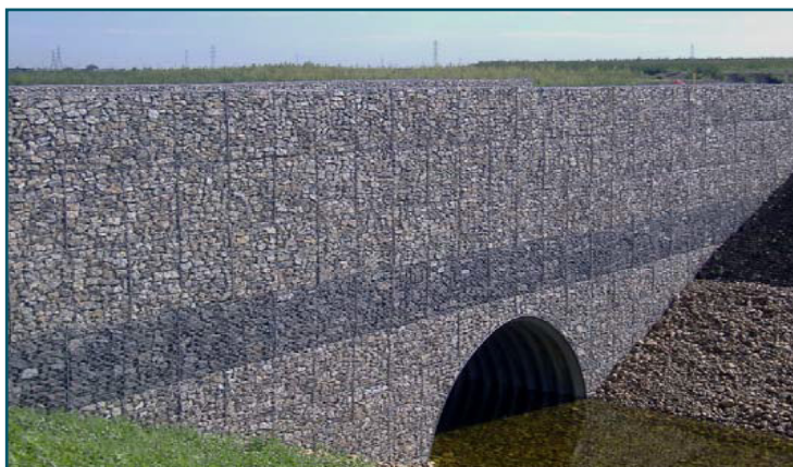
Typical Gabion Application
