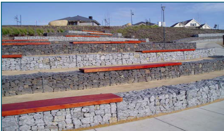
Typical Gabion Application
