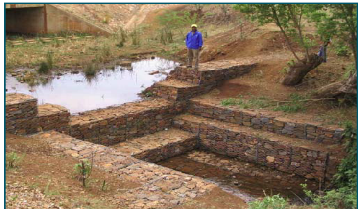
Typical Gabion Application
