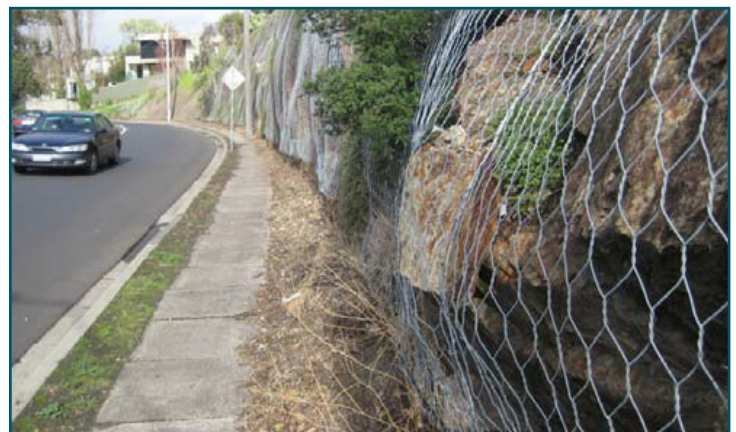
Typical Rockfall Netting Application
