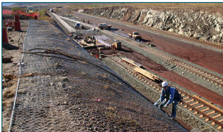
Typical Rockfall Netting Application
