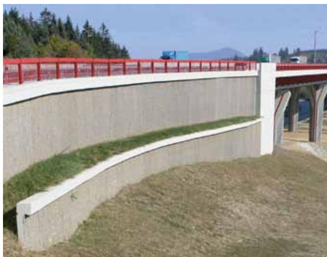
A variety of panels and finishes can be applied with either pre-cast or cast on-site panels.
