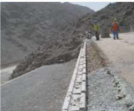
Costs are kept to a minimum with Tensar's unique modular block system which can be simply built without cranes or propping.
