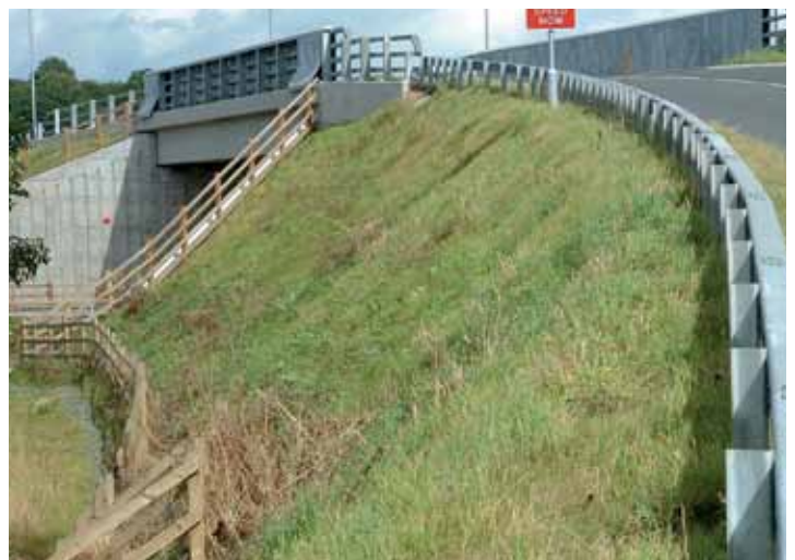
The system allows shorter construction times and reduced traffic disruption.
