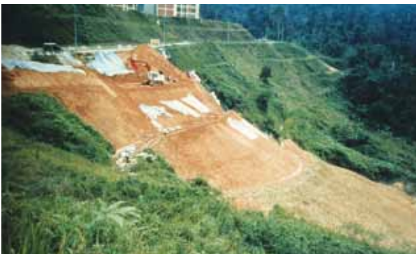
TensarTech SlipRepair System minimises off-site disposal of soil and the import of fill.
