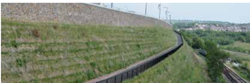
By selecting vegetation to suit local conditions TensarTech GreenSlope soon begins to establish its green face.
